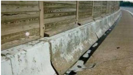
Grey concrete road barriers painted white. Illustrates the safety hazard and additional costs needed for repainting the road barriers.
