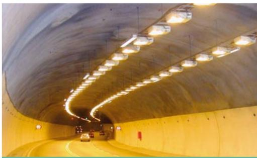
Application of white cement-based panels reduces need for lighting in underground tunnel.
